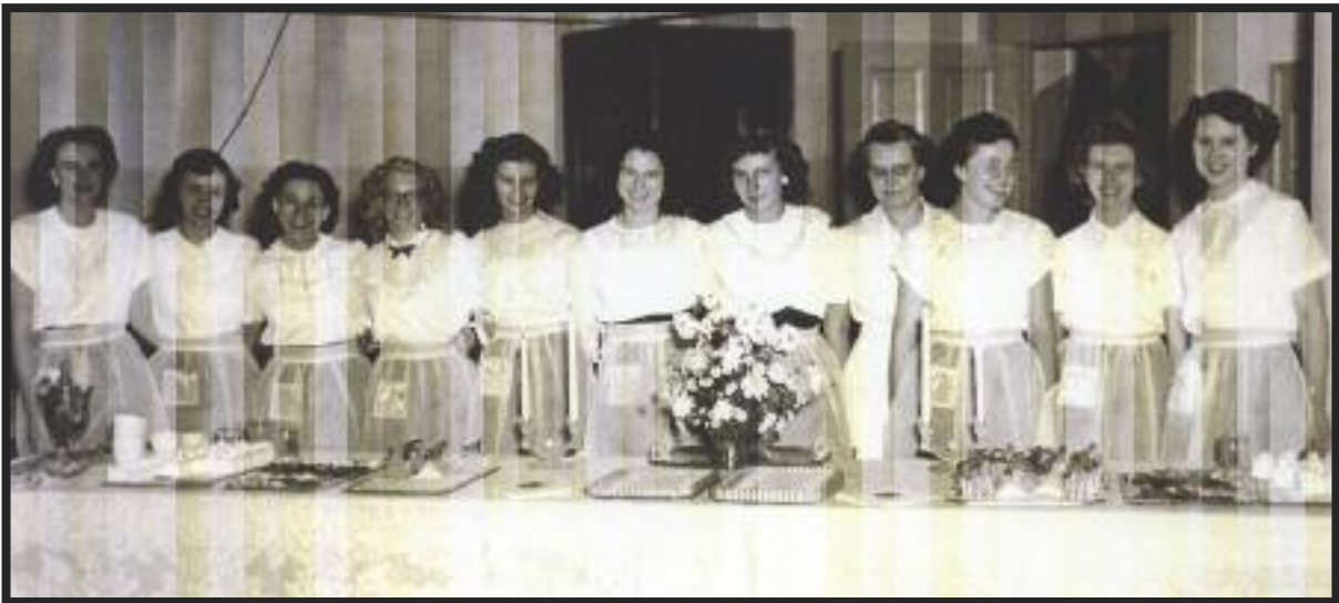
No. 81 Community Building Basement, Wedding Reception, 1949
