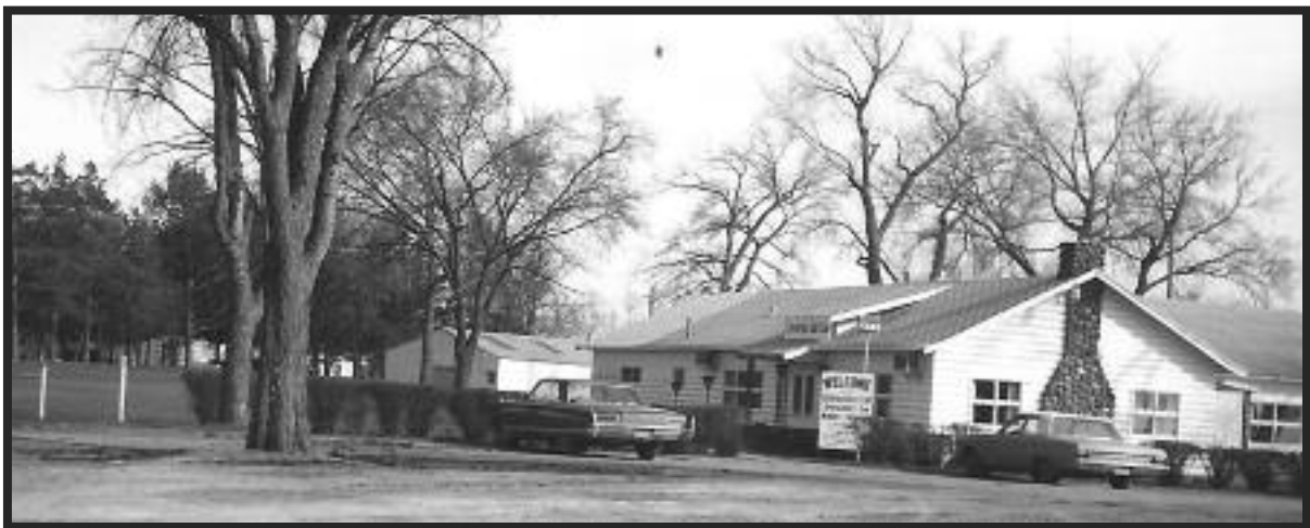
No. 95 Litchfield Golf Clubhouse
