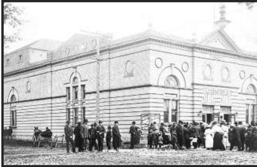
No. 70 Litchfield Opera House, 1908
