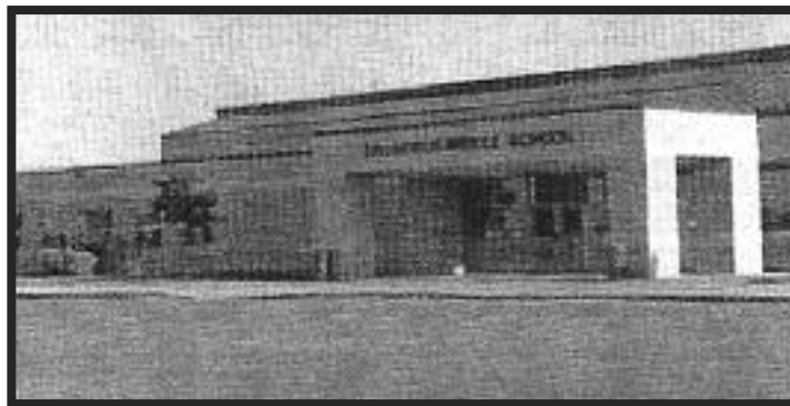
No. 60 Middle School Addition
